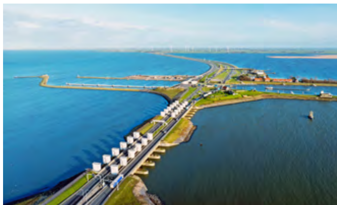
Kornwerderzand is a sluice and lock complex on the Afsluitdijk, originally built in the early 1930s and now being upgraded to help manage water levels and protect the Netherlands from flooding as sea levels rise. Projects of this kind are representative of the flood protection and water management infrastructure financed by Dutch water authorities through NWB Bank's Water Bonds.
