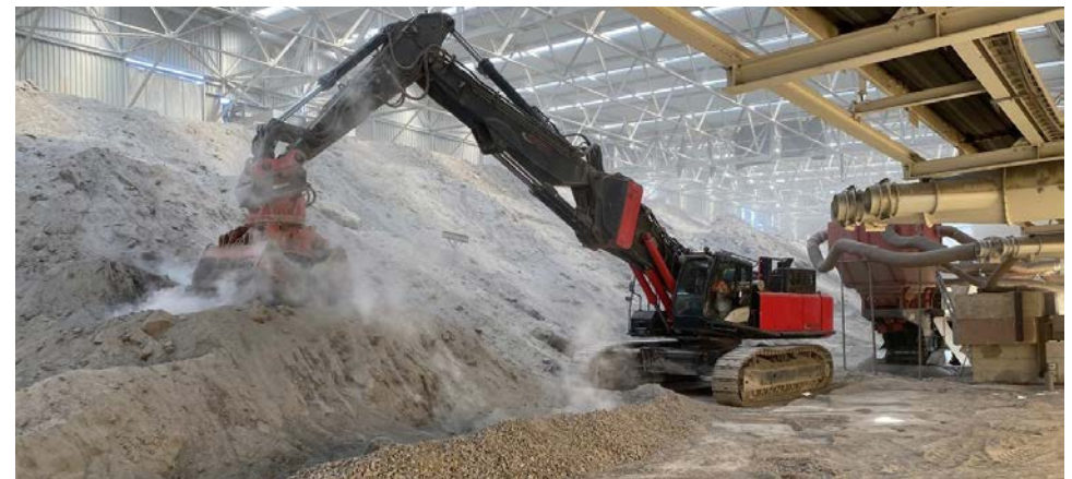
Insight into the clearance of the landfill site, which is protected from the weather by a semi-mobile roof. © BALSA GmbH
