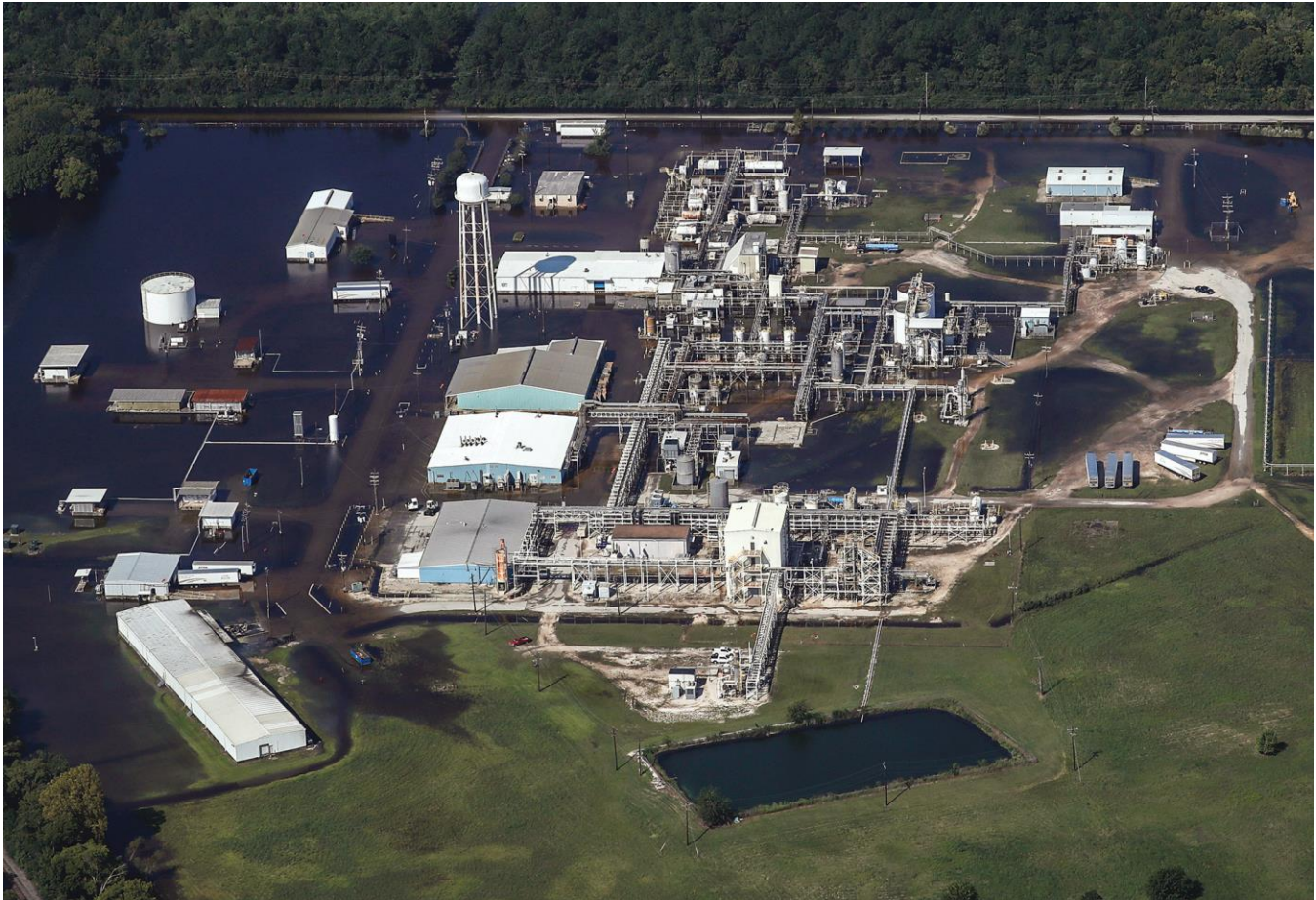
August 31, 2017, Flooding at Arkema's Houston Plant After Fire Outbreak
